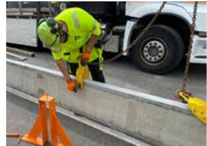
Once the element is standing on the ground, undo one of the lifting clamps. The crane will ensure the lifting chain in the remaining lifting clamp is held taut.
