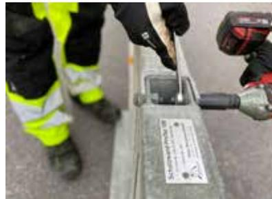
Place the support stand in the square hole which held the first (now removed) clamp and tighten the locking pin. The crane can now release the tension in the chain, and the second clamp can be removed. The first element is now standing in a stable position, and installation can be continued.
