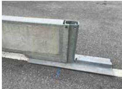
Place a start/end element on one side of the pillar and, with the aid of a crane, lift an element into position on the other side of the pillar.
